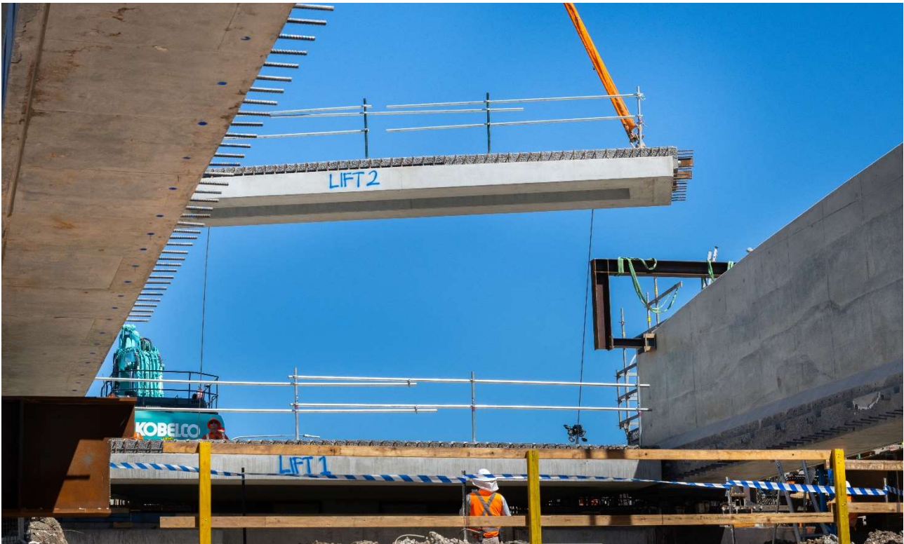
Figure 8 – Lowering of 1 st precast plank in position
