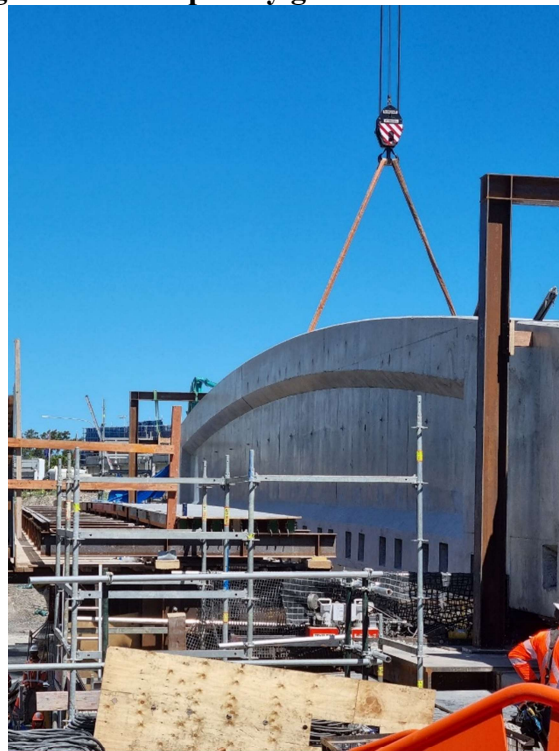
Figure 14 – Photo of the girder restraint system on site
