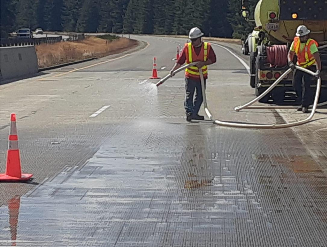
Picture 2 – Activation of Bio-based Modified Waterproofing with water
