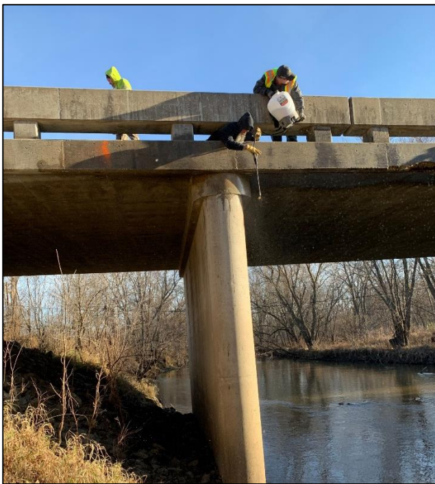
Picture 3 – Vertical Application of Bio-based Waterproofing
